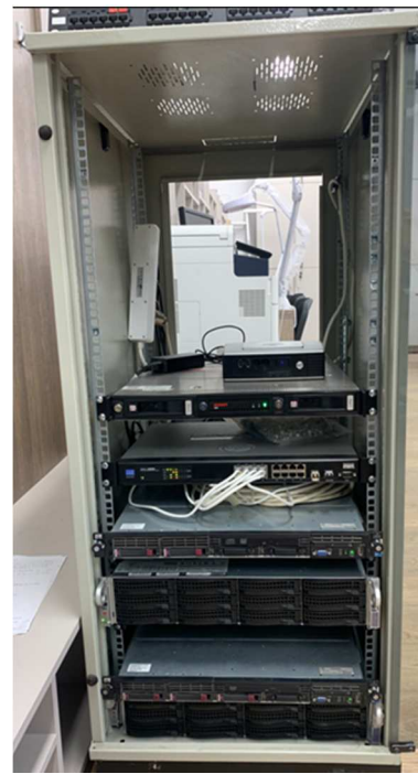
Fig. 5. Server solution and virtual machines for Janitza devices monitoring.
