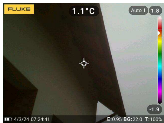
Fig. 11. The eaves area on the southern side of the analyzed building 1.
