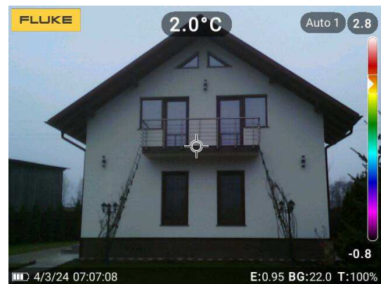
Fig. 1. The eastern part of the analyzed building 1.
