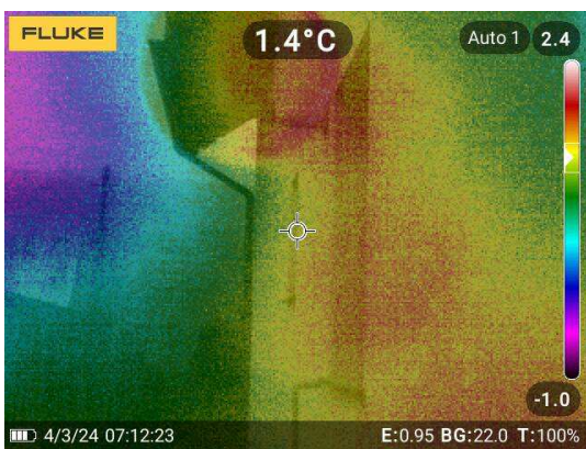
Fig. 7. The northern side of the analyzed building.
